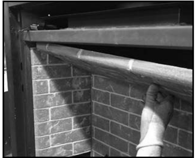
Figure 11.4 Install Top Refractory Panel
