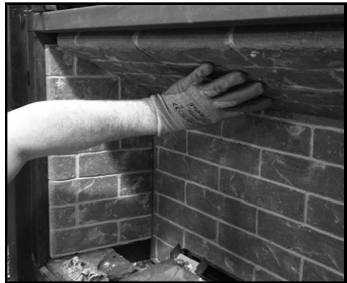
Figure 11.5 Install Right Refractory Panel
