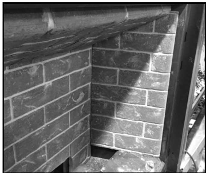
Figure 11.6 Right Refractory Panel Installed
