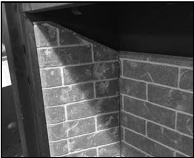
Figure 11.3 Install Left Refractory Panel
