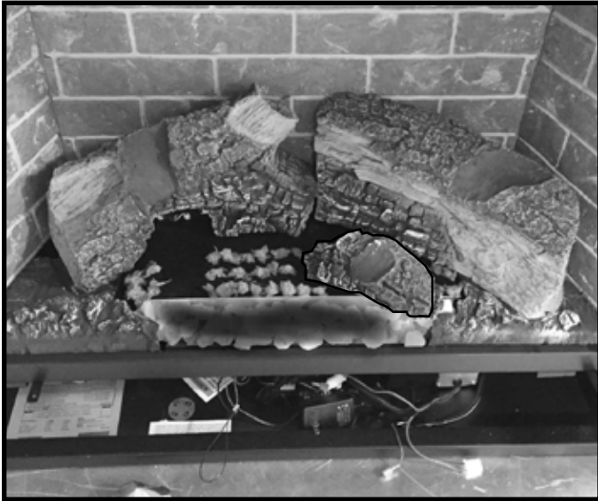
Figure 6. Burner Log Installed
